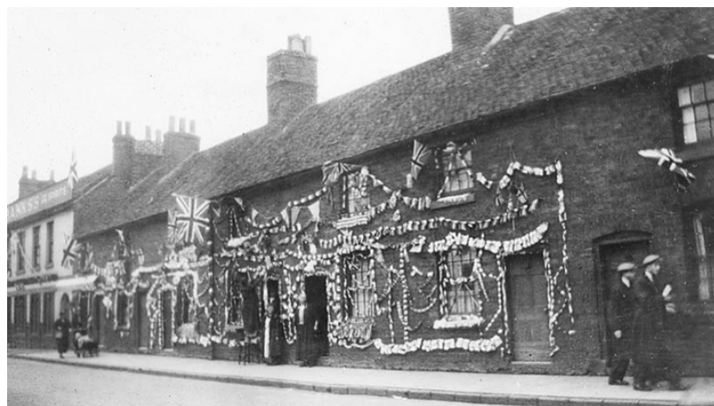
(14) Part of Woodfield Row (22-45 Bewdley Street. These date from before 1835
