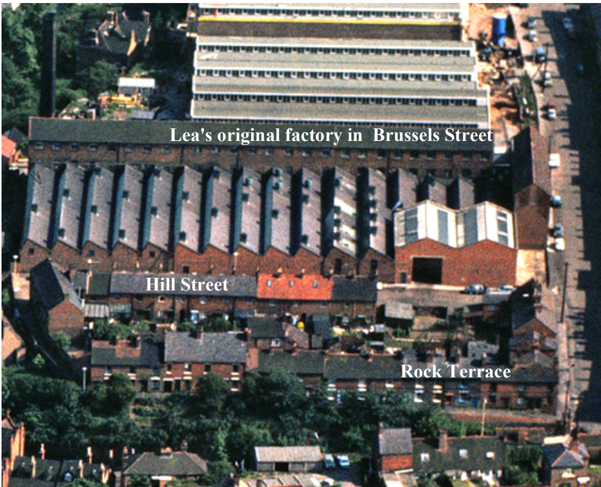
A later aerial view of Hill & Brussels Street 1967. The original 1801 Lea's factory is seen bordering Brussels Street with north light weaving sheds added towards Hill St since 1897. Courtesy Kidderminster Past.
